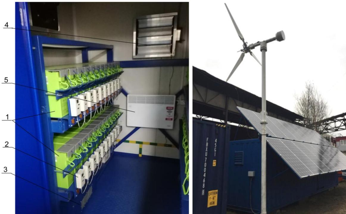
**Fig. 6. An experimental model of a combined energy storage unit installed in a wind photo-diesel power complex:**
